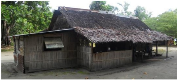
Figure 1 A traditional housing structure in Lokwitua, PNG Islands.
