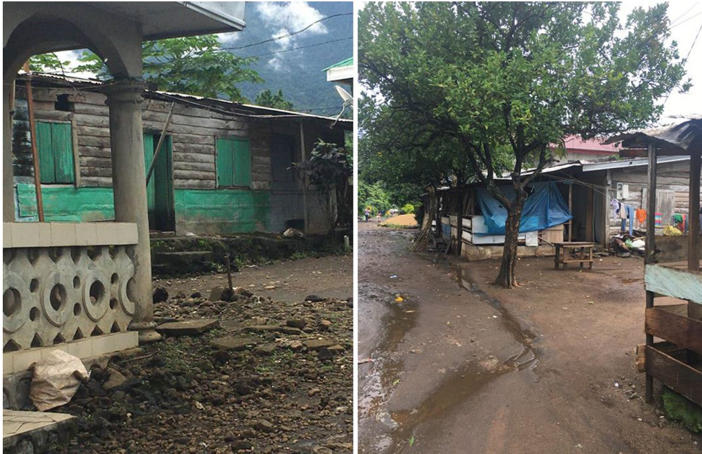
Fig. 1 Plank houses with crevices on the walls
