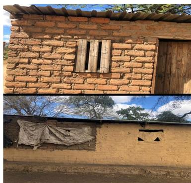
**Fig. 6** Brick houses under iron sheets with open eaves, holes and open makeshift windows at Tongogara refugee camp Zimbabwe, 2021
