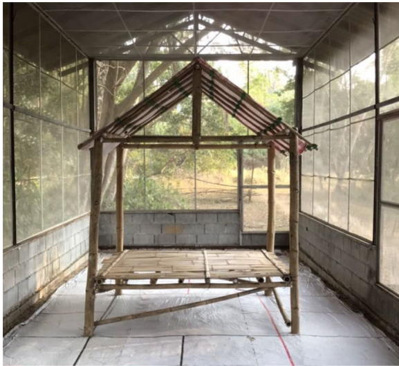
Fig. 3 Bamboo temporary, open structures at Kasetsart University (KU)
