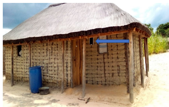
Fig. 3 Deployed ATSB bait station on residential structure
