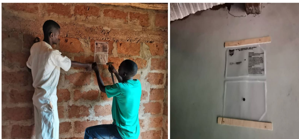
Fig. 2 Installation of Mosquito Shield™ products on home walls
