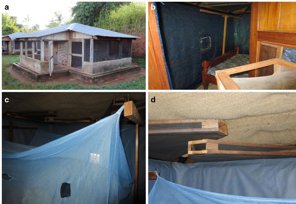
**Fig. 1** **a** East African experimental huts in Zeneti village, Muheza District, northeast Tanzania. **b** Pyrethroid ITWL (ZeroVector<sup>®</sup>). **c** Non-pyrethroid ITWL (PermaNet<sup>®</sup> Lining) + LLIN (Interceptor<sup>®</sup>) with eaves partially blocked. **d** Eave baffles and hessian sack cloth ceiling
