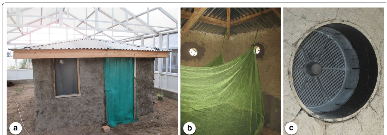
Fig. 1 a Experimental house ( 3 \times 3 m) inside screen-house with mud wall, corrugated iron roofing, screened window and door. b Inside the house with untreated bed net, sealed eaves and eave tubes. c Eave tube with treated insert as seen from the outside
