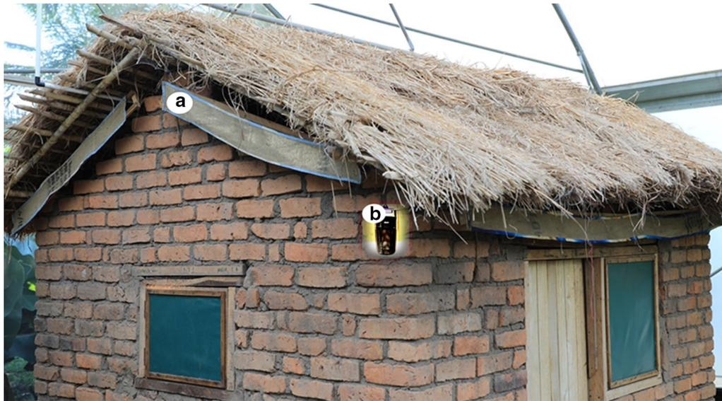
**Fig. 2** Illustration of transfluthrin-treated eave ribbons wrapped around the eave space (a), and Mosclean trap (b). In this study, the Mosclean trap was used as an intervention and was placed always indoors. A separate indoor sampling trap, CDC-light trap was used for measuring efficacy of intervention. The eave ribbons and traps were assessed individually, or in push–pull system by putting them in the same houses or adjacent houses
